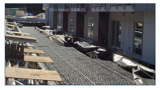
This site came with several challenges; the first was that the tank location needed to be installed in a tight space with height restrictions. Secondly, the tank location was built in an existing, irregular-shaped planter courtyard. This made the tank more difficult to fit into this unusual space, but we were able to find a tank configuration that fit well and maximized the available space.
