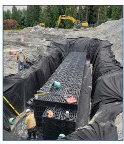
The project began with EcoBloc Maxx base plates laid at the base of the site bed and secured with connector pieces. Blocks were then stacked and connected up to five layers and finished further endplates and pipe connections. Pipe adapters were used to secure the pipe connections in place. The structure was then wrapped with 8 oz. geotextile and an inspection port was secured. Finally, the site was backfilled evenly with gravel.
