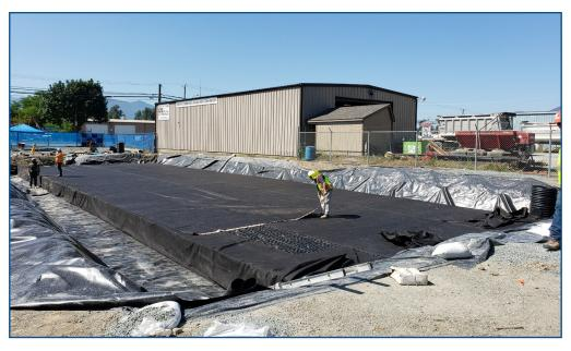
This site required increased onsite storage required by the Municipality, high water table & constant heavy traffic loading on the tank. We used the Graf EcoBloc Maxx block to create this  $240~\text{m}^3$  detention tank, complete with accessories like the manway extension in the photo below.
